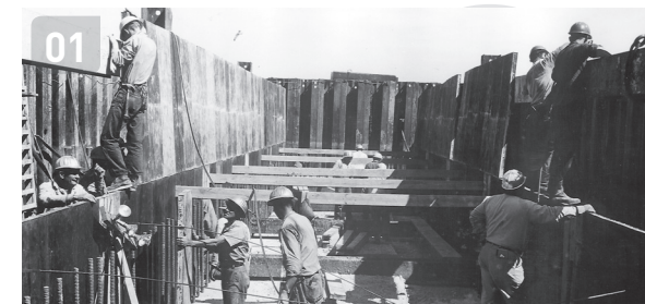
Construction of the Hart Bridge, connecting downtown with the Southside
