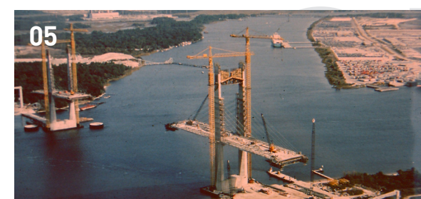
Construction of the award-winning Dames Point Bridge underway in the late 1980s
