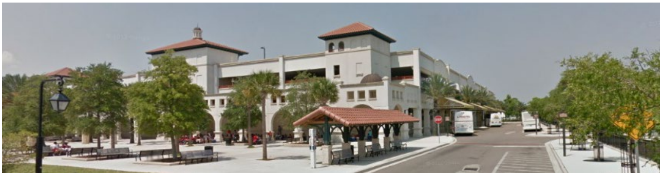
Photo 20: St. Augustine Historic Downtown Parking and Transfer Facility
