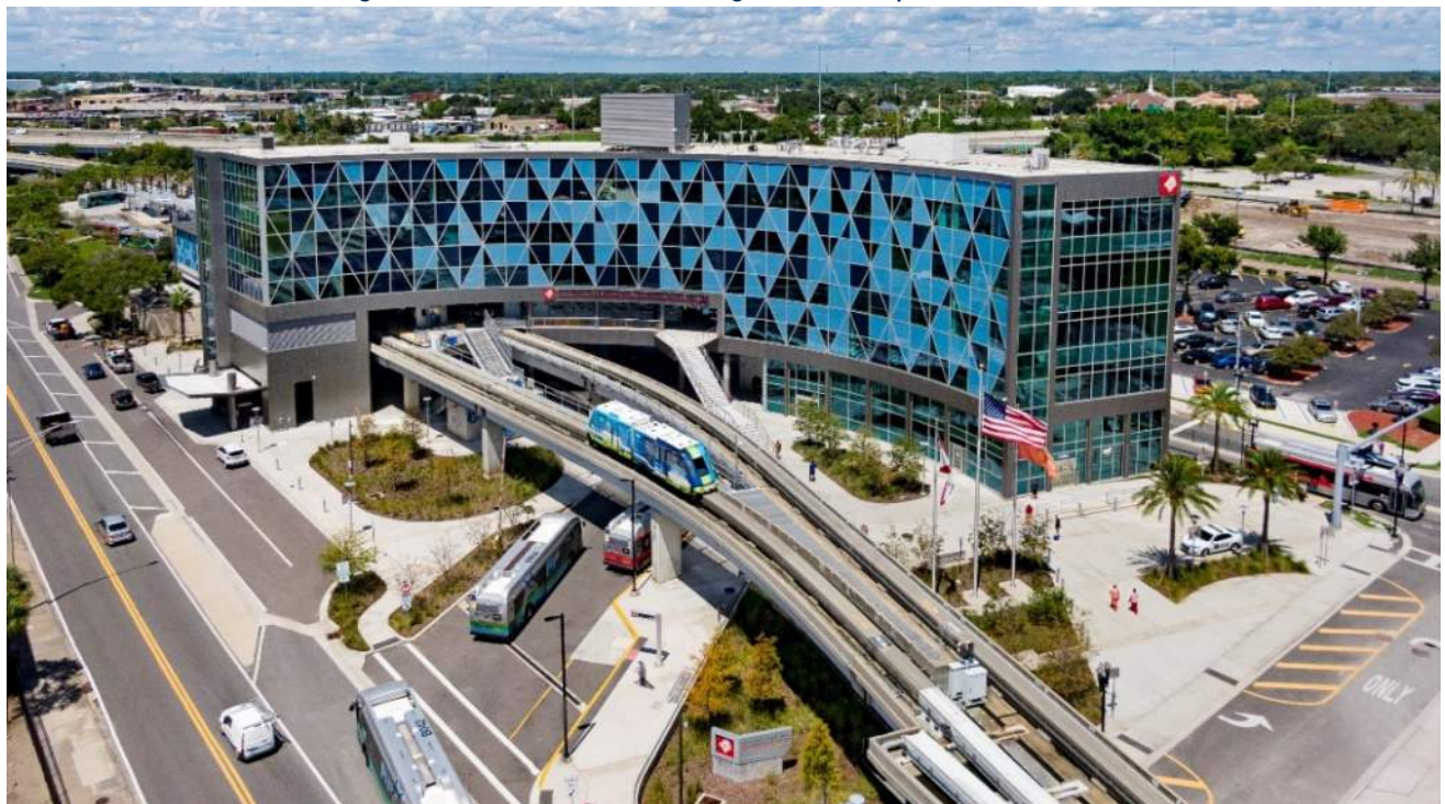
Figure 9. The Jacksonville Regional Transportation Center
