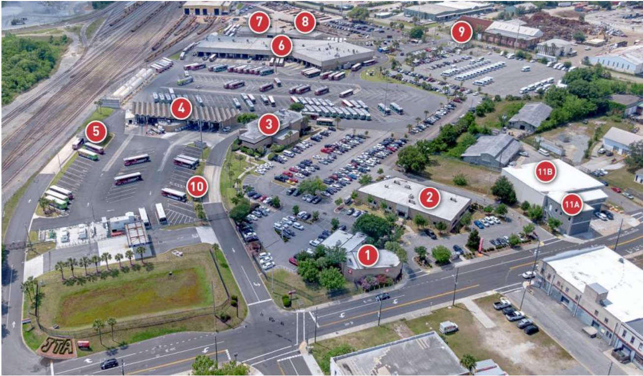
Figure 5. Myrtle Avenue Operations Campus
