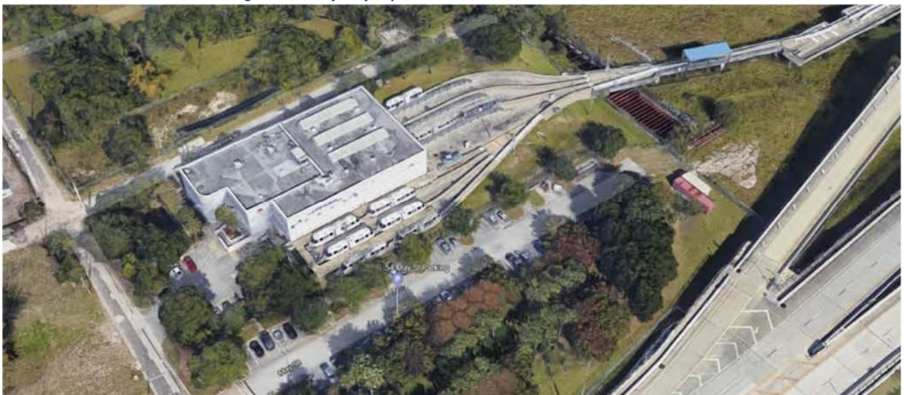
Figure 11. Skyway Operations and Maintenance Center
